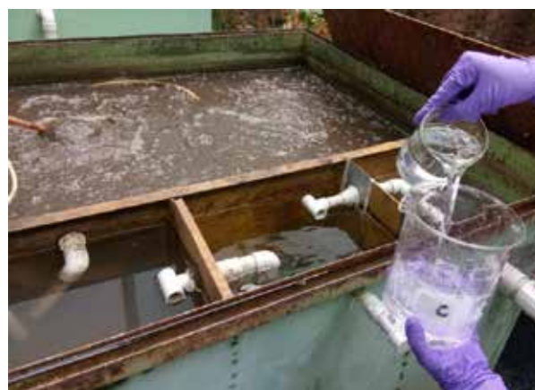
Clear water from canteen wastewater after treatment
