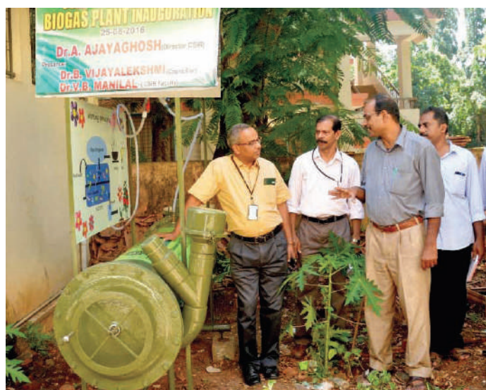
Installation of NIIST biogas plant at Govt. UPS, Poojappura
